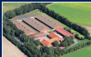
KI station Saerbeck KI station Kiebitzheide Lengericher Damm 23 48369 Saerbeck Tel. +49 25 74 93 74 21 Fax +49 25 74 93 74 50
